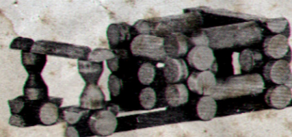
FILLING STATION (Roof Removed)
